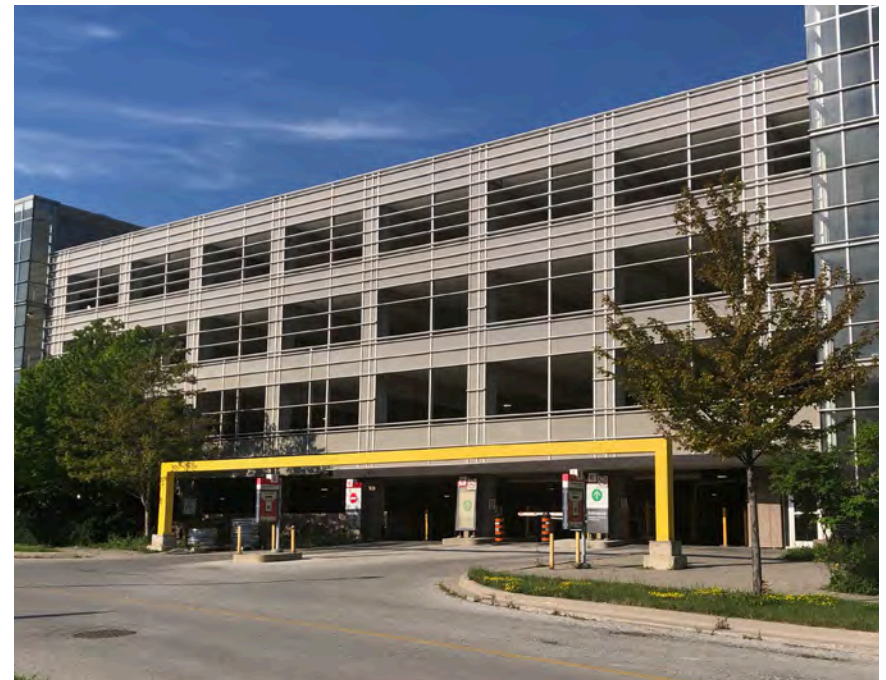
Entrance to the Student Services Parking Garage on James Gilles Street.
